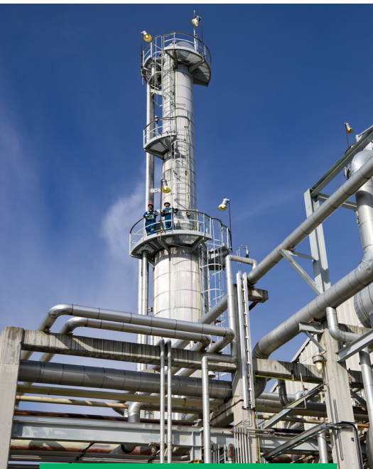
Waterton Gas Complex
