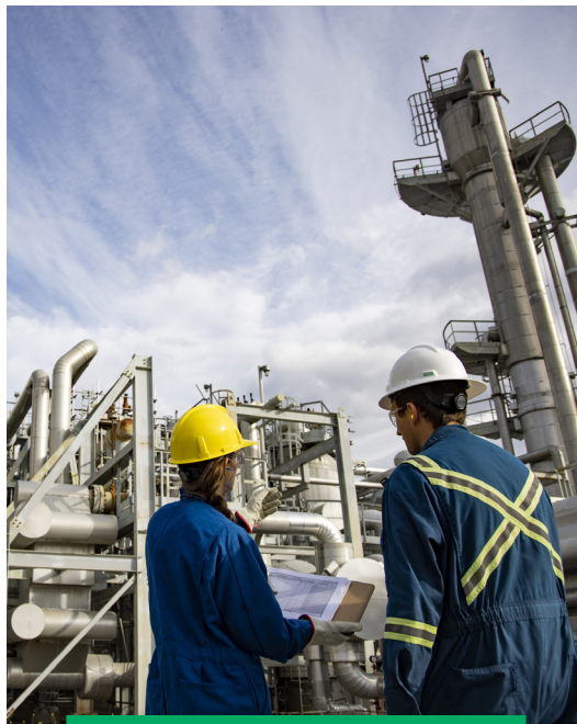
Jumping Pound Gas Complex
